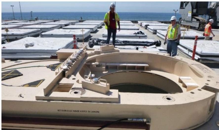
1 This photo shows the vertical cask transporter being aligned to the mating device,
